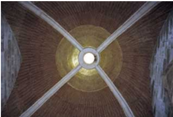
Ceiling of church
